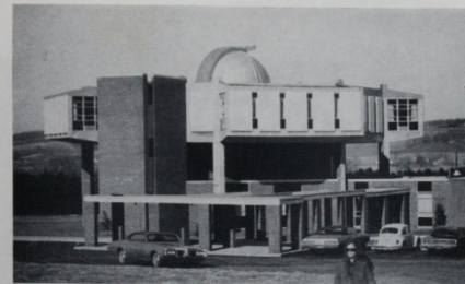
The Gruber-Knedler Planetarium and Observatory has the star theater on the first floor, requiring considerable height (shaded section), and the telescope dome on top. This and the other circular wing of the Grim Science Hall are connected by the lobby seen partially at lower right.
